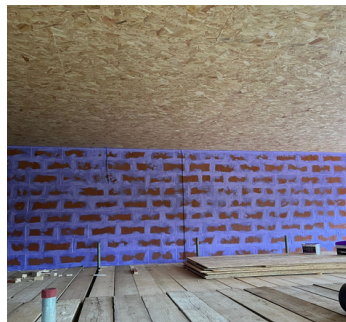
Passive Purple Brush applied to wood fibre.
