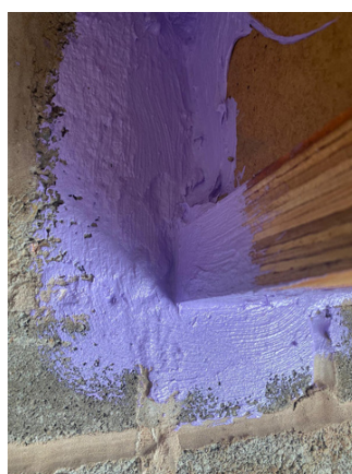
Joist connection on to masonry wall.
