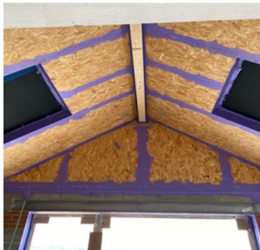
OSB board connections.
