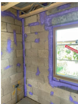
Internal brick connections.
