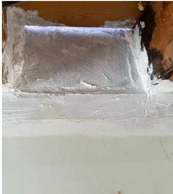
Joist connection in masonry wall using Airtight White Brush.
