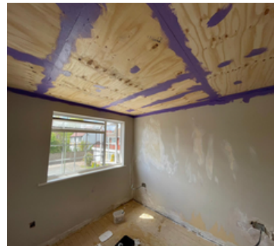
Plywood connections.
