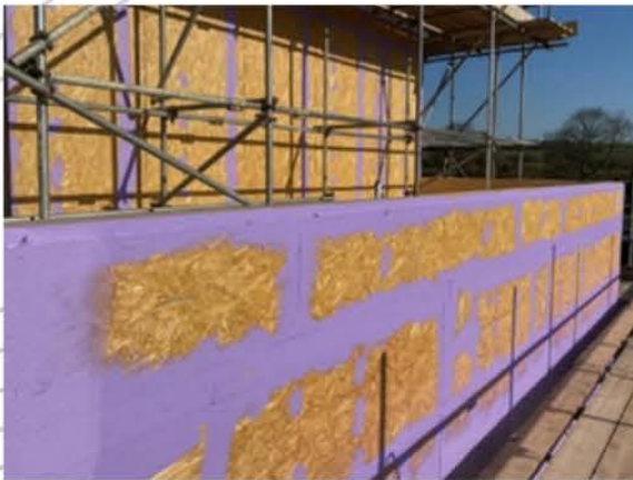
5.1.5 Preparing board joints before the application of Passive Purple External.
