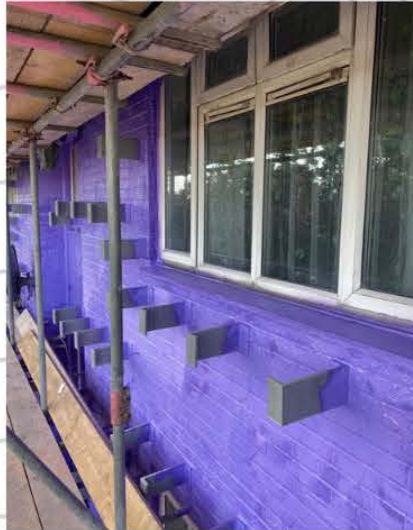
5.1.3 Helping hand brackets painted with Passive Purple External Brush.
