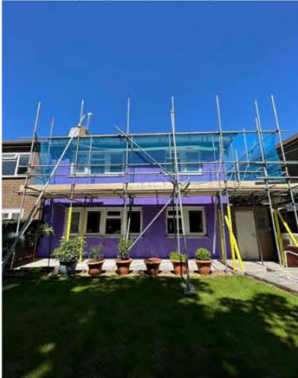
5.1.2 Retrofit at the rear of property.
