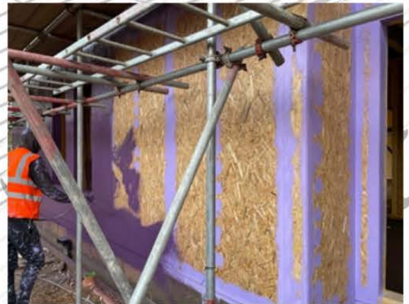
5.1.6 Prepared wall connections before the application of Passive Purple External.
